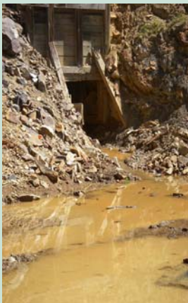
Above: The adit of the Standard Mine at Level 1 is shown in the background.
